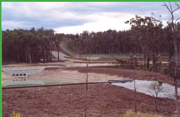
E Rosion Retention Pond & Scour Protection Mat Newstan Mine
