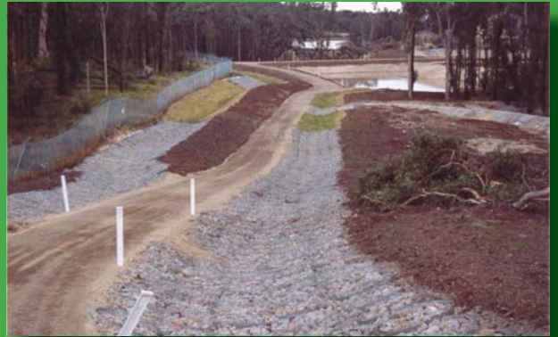
E Rosion Drainage Channels to Retention Pond Newstan Mine
