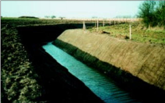
Completed channel section during the germination process.
