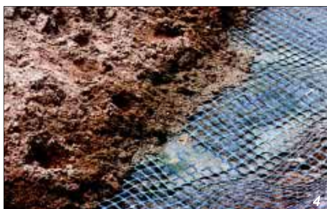
Photo 4: The geogrid apertures allow the soil interlock and full transfer of high tensile forces.
